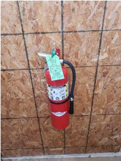
16 Administration and General Add new extinguisher in kiln shed
